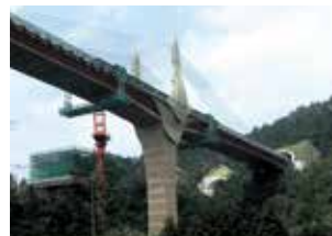
栗東橋(滋賀県大津市) Ritto Bridge (Shiga)
