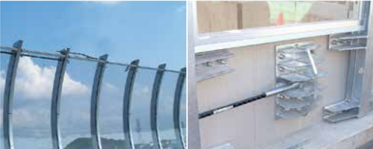
遮音壁落下防止装置 Noise insulation and wall dropping prevention device
