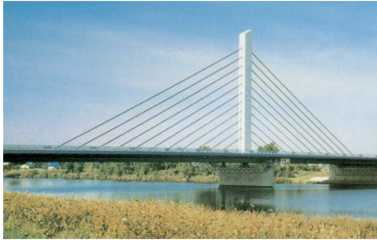
BAN-NAGURO BRIDGE (HOKKAIDO)
