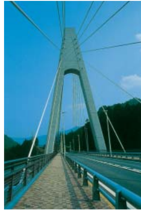
OKUTAMA BRIDGE (TOKYO)
