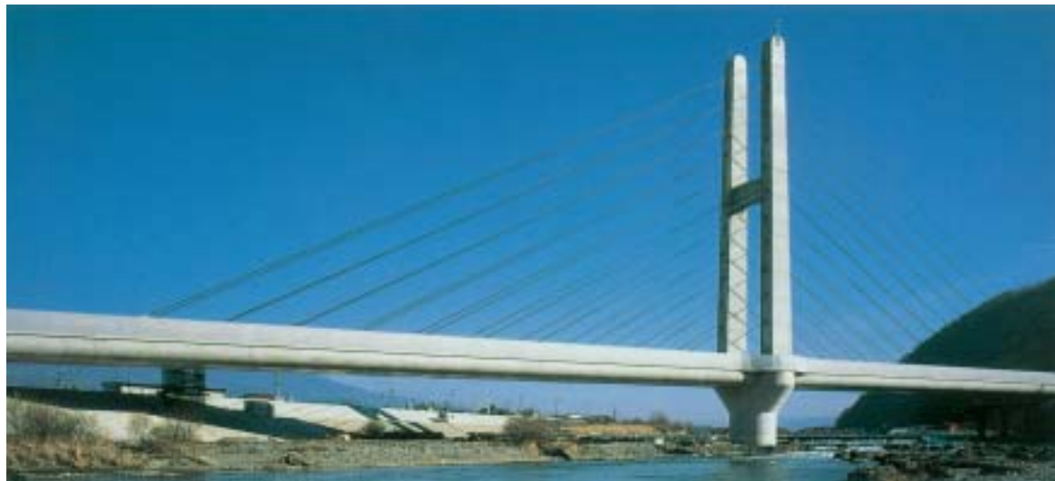
DAINI CHIKUMAGAWA BRIDGE (NAGANO)
