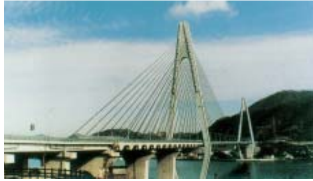
IKUCHI BRIDGE (HIROSHIMA)
