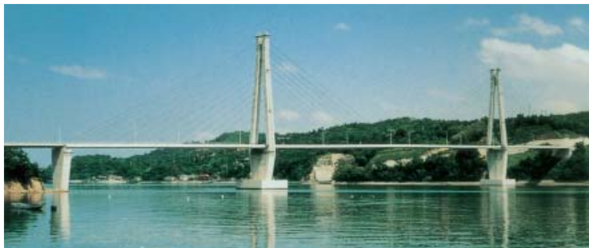
OHSHIBA BRIDGE (HIROSHIMA)
