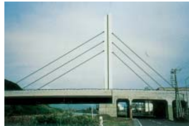
RURUMOPPE BRIDGE (HOKKAIDO)
