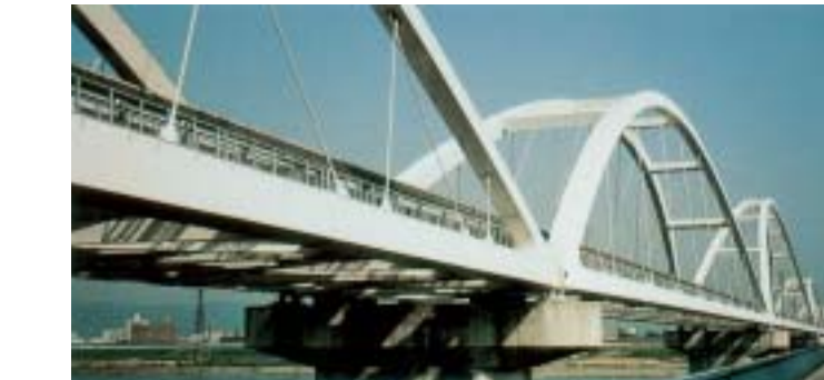
OSAKA MONO-RAIL BRIDGE (OSAKA)
