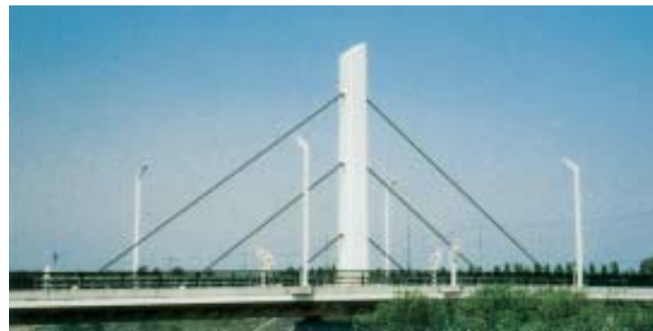
MAEDA SHINRIN KOEN BRIDGE (HOKKAIDO)
