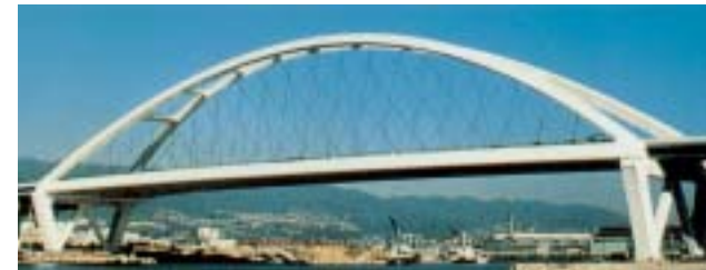
NISINOMIYA-KO BRIDGE (HYOGO)
